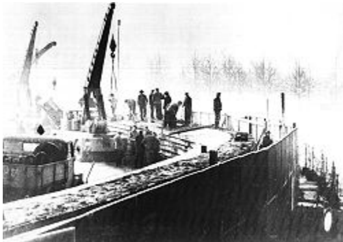
East German construction workers building the Berlin Wall, November 20, 1961.
